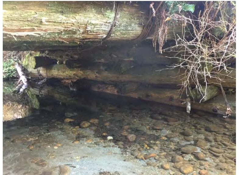
Left Bank Abutment when facing downstream
