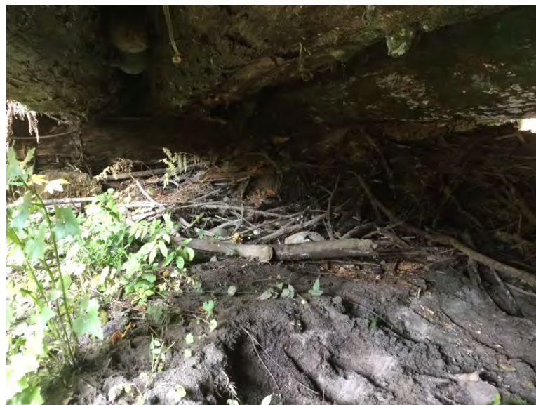
Right Bank Abutment when facing downstream
